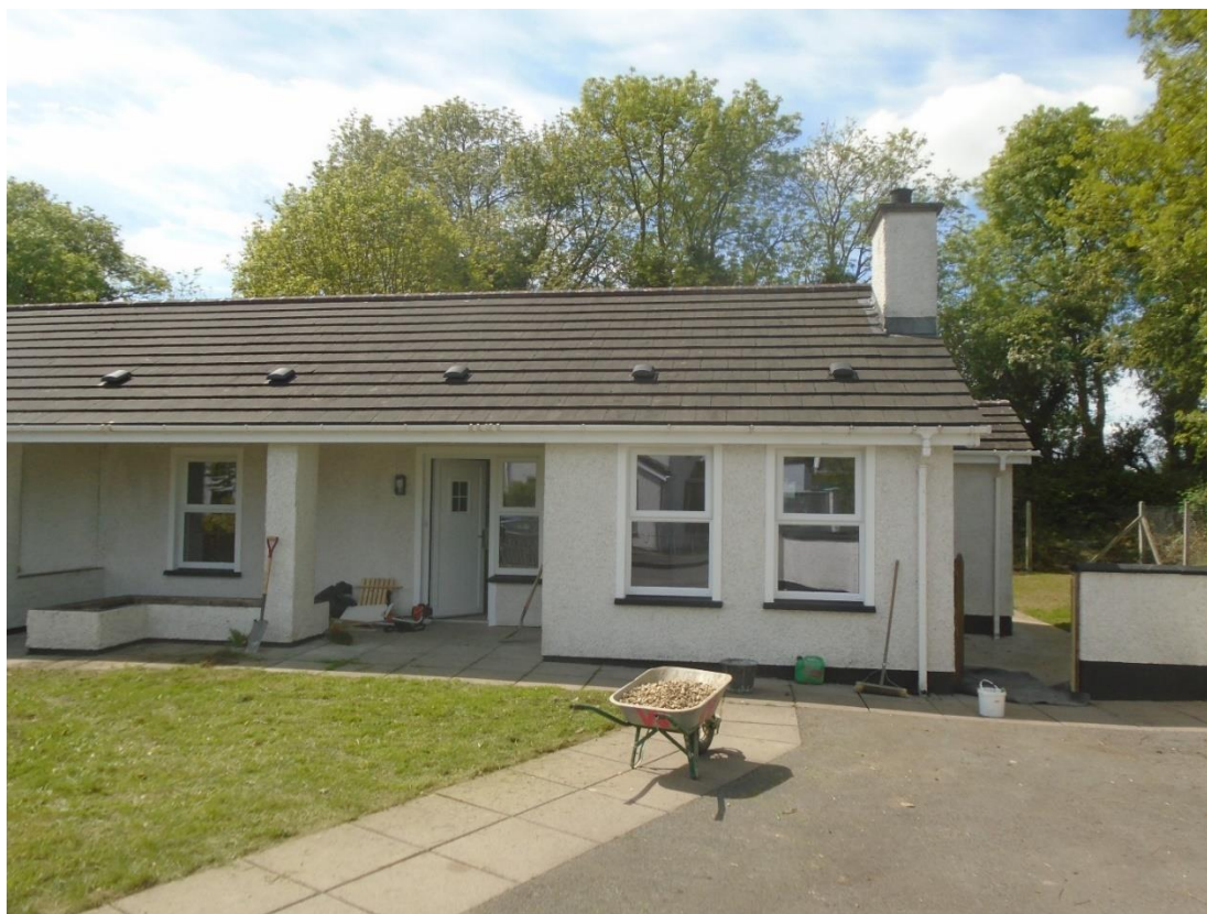
Upgrade works ongoing at Local Authority bungalow.
