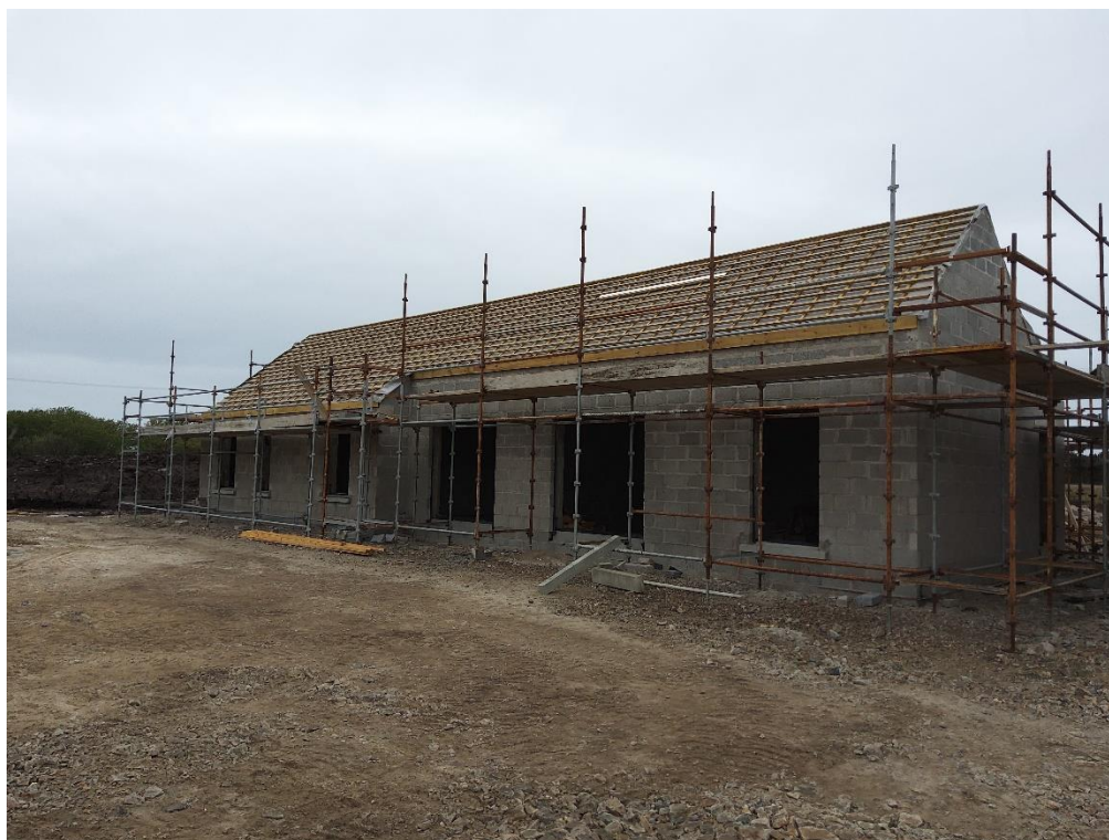
Donegal Parents & Friends – Group Home Project Dungloe – Under Construction.
